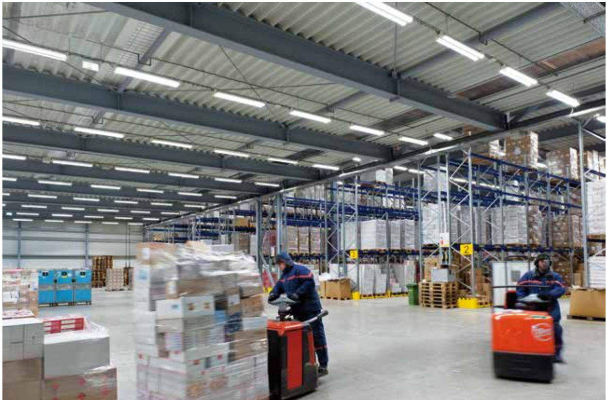
► NORKA luminaires for extreme temperature areas; here -25 °C in a cold storage
