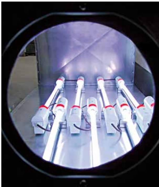
➤ NORKA luminaire NEUSTADT with T-UV-C lamp for disinfection in air filter system
